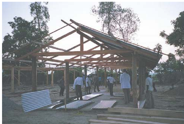
'Long-house' building capable of sheltering five to six families
